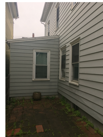
EXISTING CONDITION PHOTO #4
