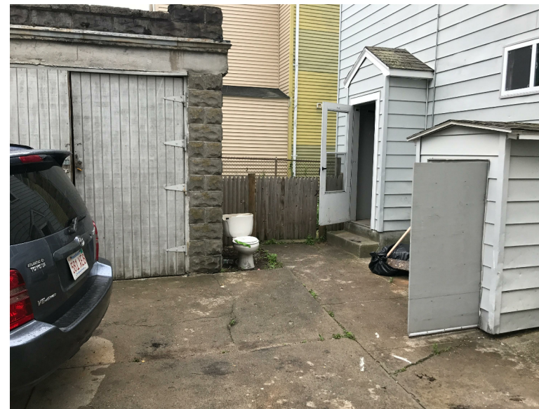
EXISTING CONDITION PHOTO #3
