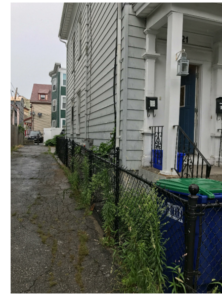
EXISTING CONDITION PHOTO #2
