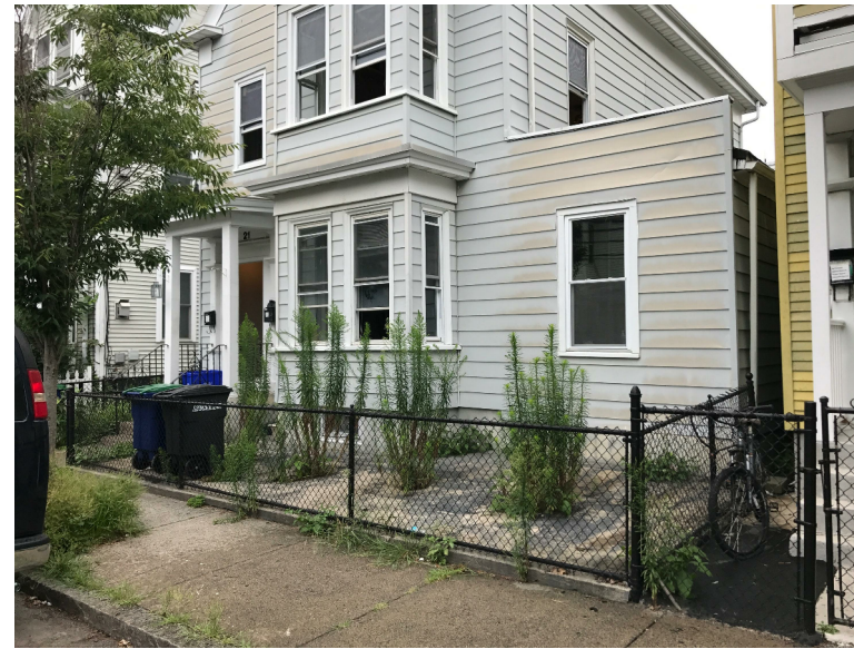
EXISTING CONDITION PHOTO #1
